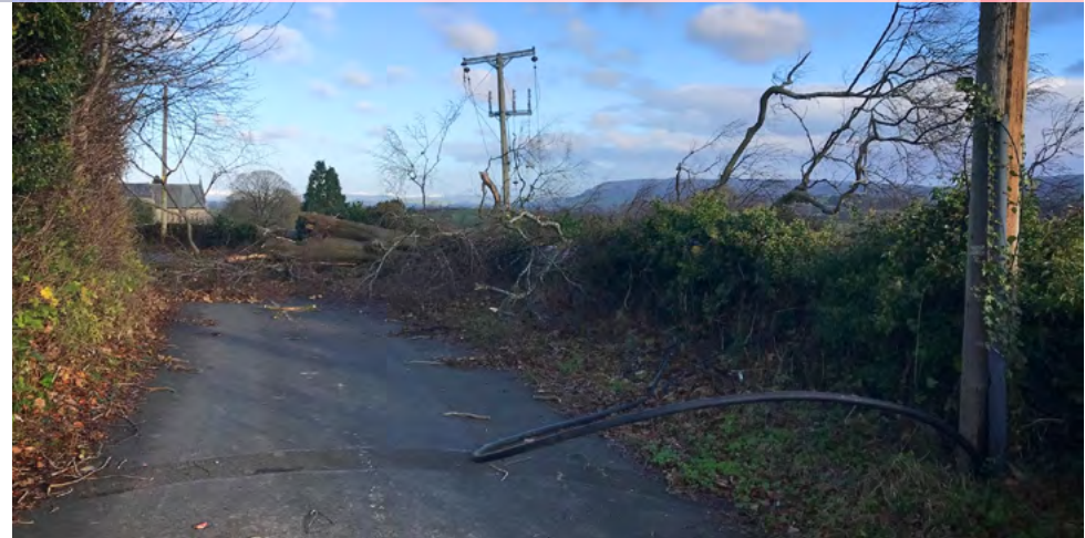
Storm Arwen 27 Nov 2021 Image supplied by Electricity North West)
