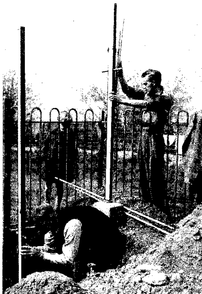
Levelling at an opened fundamental bench-mark, constructed before World War I.
