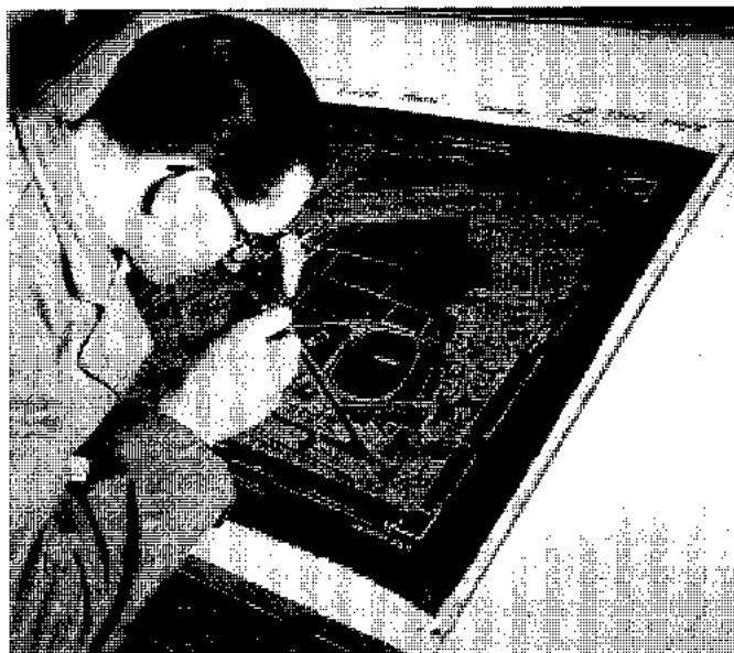
Photowriter working on a negative of a large-scale map.
