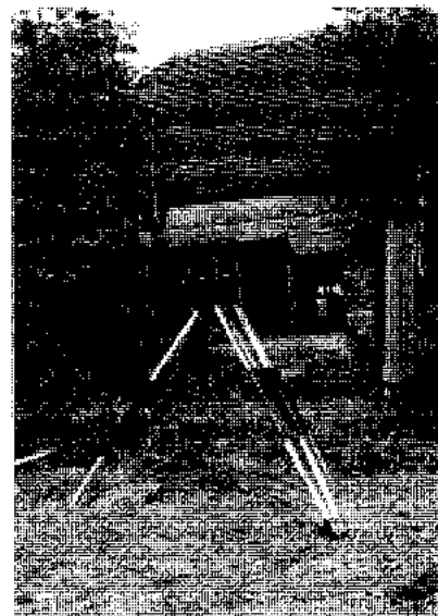
Odson's Barn. This obstructed the line of the Ridgeway base, and it was necessary to remove the sides to measure through it.
