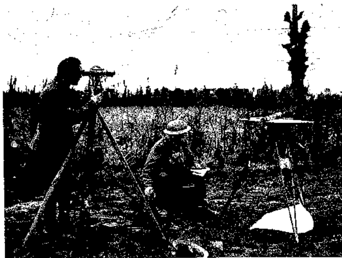
Use of Lucas daylight signalling lamp for triangulation. The telescope and plane-table were used to obtain a rough alignment.
