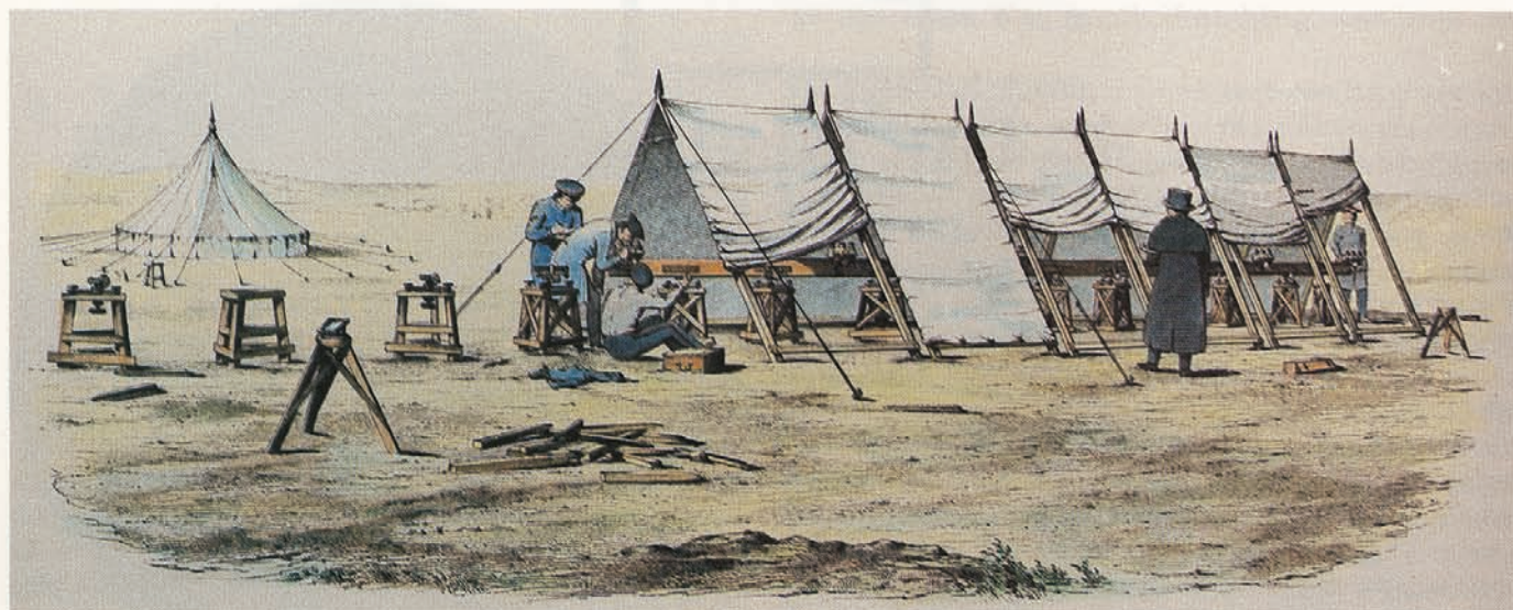
'Sketch shewing the mode of proceeding in measuring the Lough Foyle Base'.
